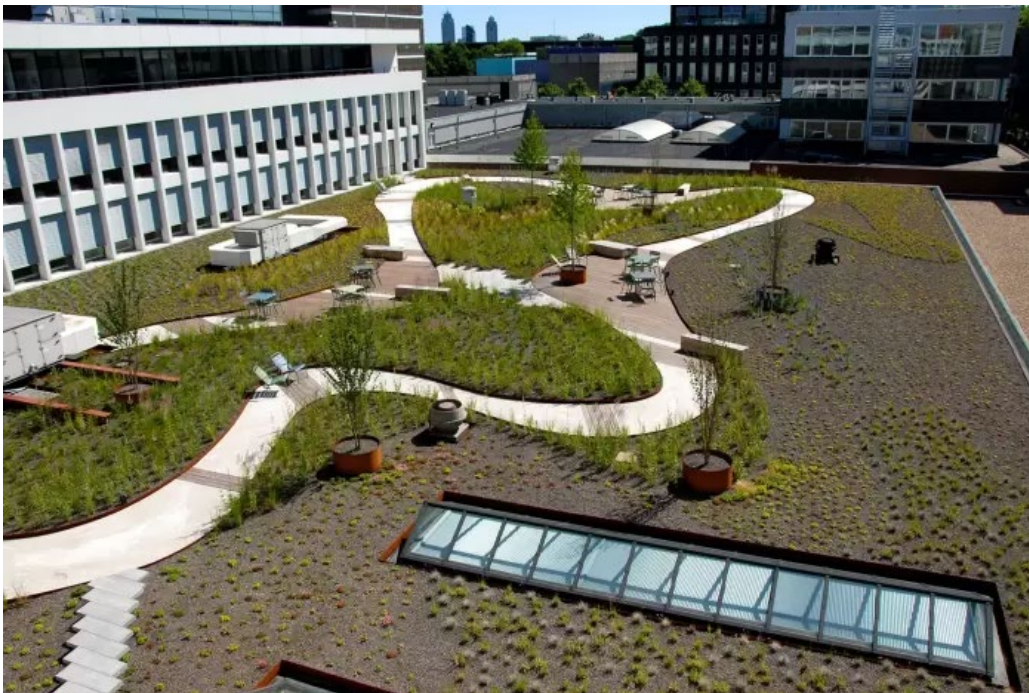
Multifunctional roof with a polder function (water control) in Amsterdam's Zuidas business district.
